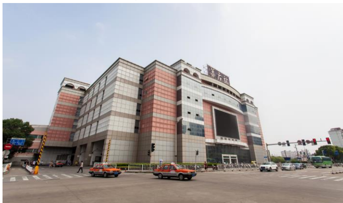
Current Xinzhuang Metro Station
